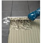
standard set adhesives. If fixing a stone showertray, this too should be fixed using tile adhesive as above, taking care to ensure that the tray is correctly aligned and level. Once the showertray has been fixed then floor tiles can be laid up to the showertray.
